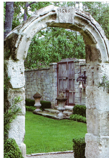
ROOM TO EXPLORE: A circa-1626 limestone arch, set within a Japanese yew hedge, frames the symmetrical entry to a side courtyard.
